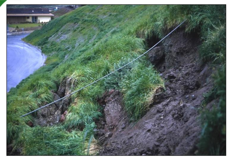
Cut slopes failures are usually shallow, involving a wet mat of organic material, which often detaches at the root line, within 1 to 3 feet of the ground surface
