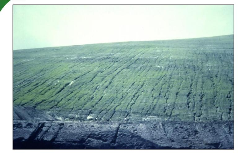
In the 1988 the old UBC an allowance was made waiving terrace drains for fill slopes inclined at 3:1 or flatter. This view shows rill erosion developed on such a slope, despite a healthy grass cover
