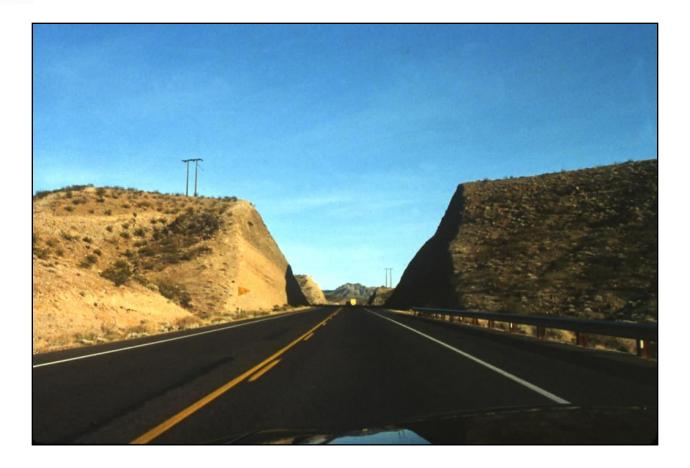
Steep cuts in competent rock may remain stable for long periods of time. Even so, a wide debris trough should be excavated at the foot of such cuts to catch falling rock and dissipate its energy.
