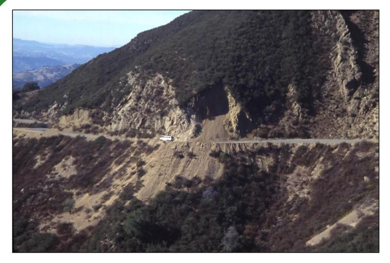
Selective raveling of steep cuts in competent rock are a recurring problem. Joint patterns and intensity generally control long-term behavior. Note the sawtooth shape of the raveling cut shown above, caused by the intersection of steeply-inclined bedding and one set of joints.
