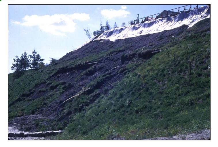
When this mat of vegetation is subjected to sustained intense precipitation, it tends to separate like a rug falling off a polished floor, as shown above.
