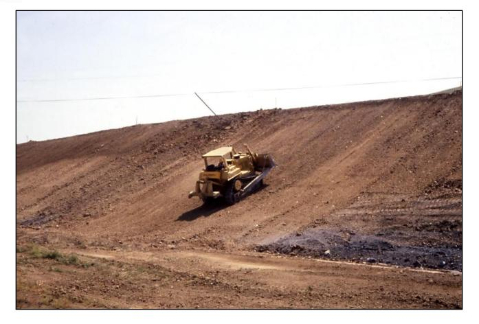
Track walking a fill slope will not compact it appreciably because the track contact pressures (between 5 and 10 psi) are well below those imparted by a mechanical compactor (>135 psi for a pad roller)
