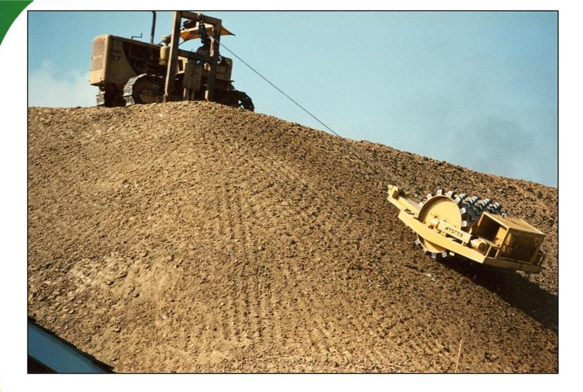
Rolling a fill slope with a pad roller imparts between 135 and 175 psi contact pressure beneath the roller teeth
