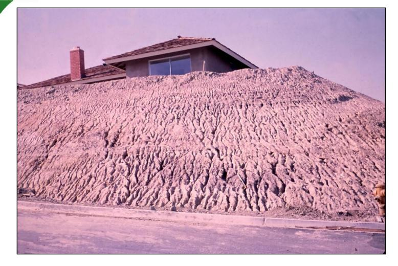
Rill erosion is common in low cohesion fill materials, like sands and silts. This photo shows the impact of a single series of storms on an unprotected fill slope
