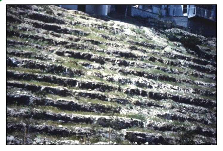
Serrated cuts", or "step cut" slopes are intended to retard rill erosion in semihomogeneous materials. They are used chiefly in semi-arid climates.
