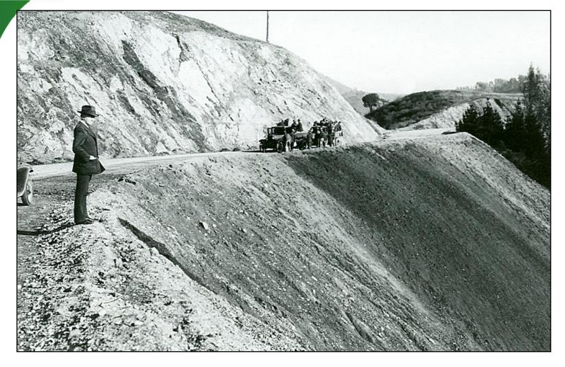
This shows a sidehill fill slope supporting a newly constructed road along the crest of the Berkeley-Oakland Hills, CA above Claremont Canyon in late 1934.
