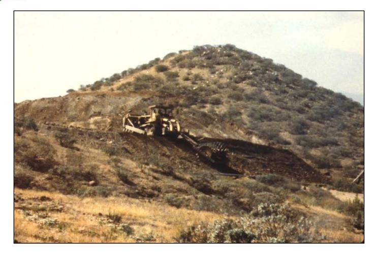
The contact pressure is the roller weight on the teeth multiplied by the cosine of the slope inclination (about 11% reduction on a 2:1 slope).
