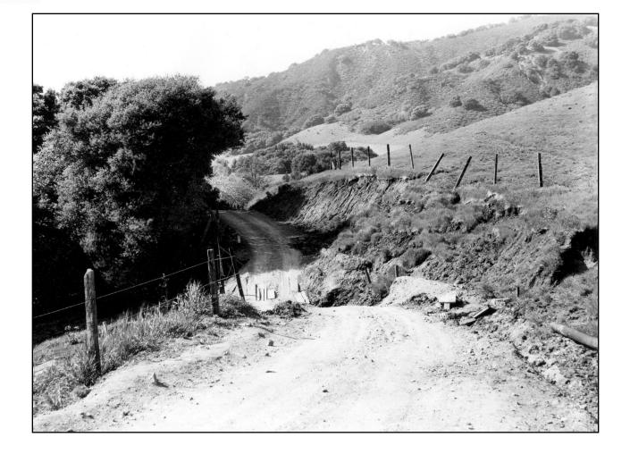
Steep cuts in weathered rock, shale or soil may degrade rapidly, especially during periods of sustained precipitation and runoff, as shown here (note tilted fence posts).
